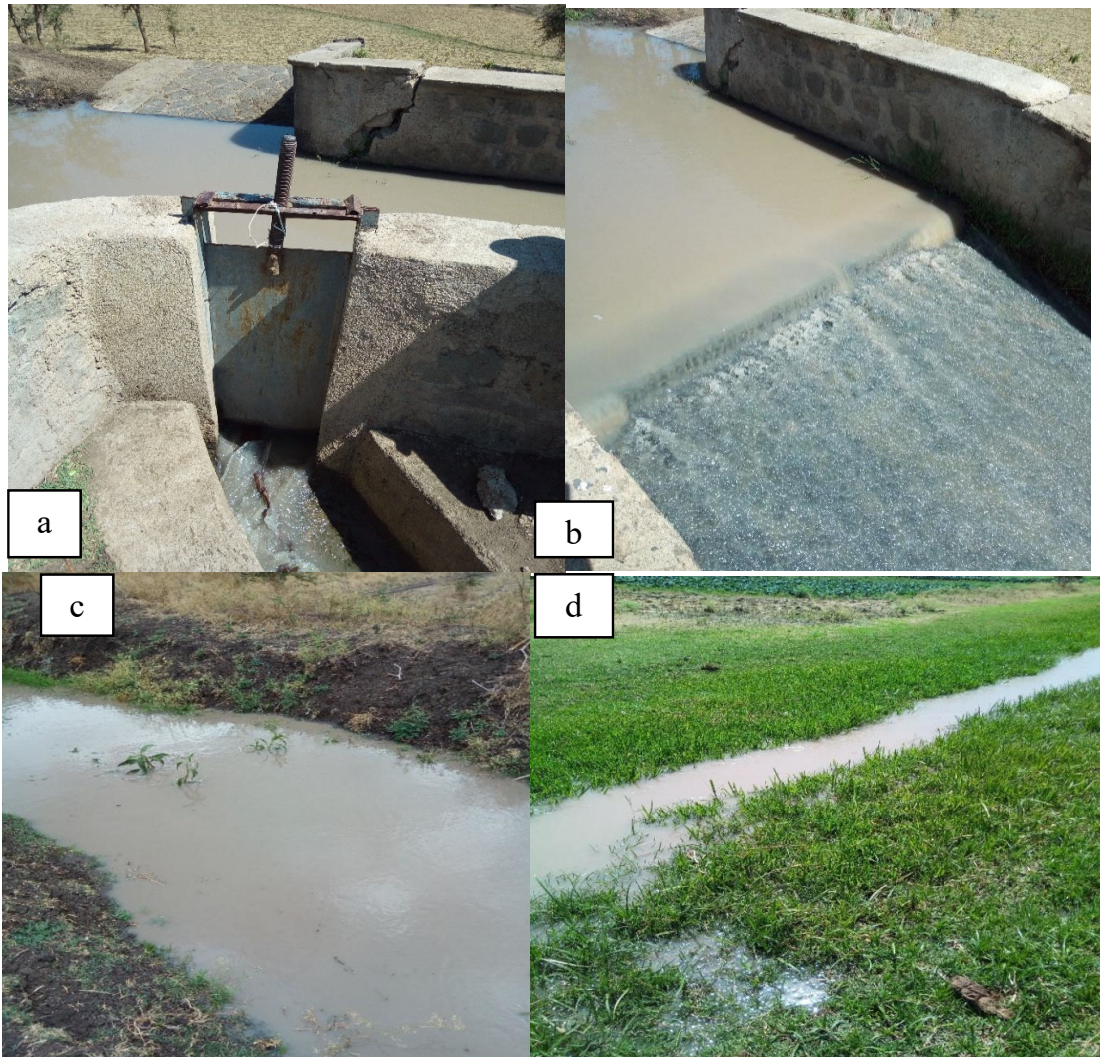
Figure 1: a, b, c and d are the Samples of the Koftu Irrigation Scheme Water Delivery Division Box and Canals
